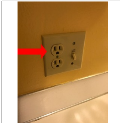
Kitchen electrical receptacle is not GFCI
