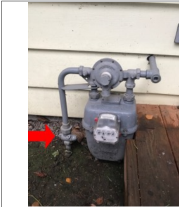
Main fuel shut off located on east side of exterior
