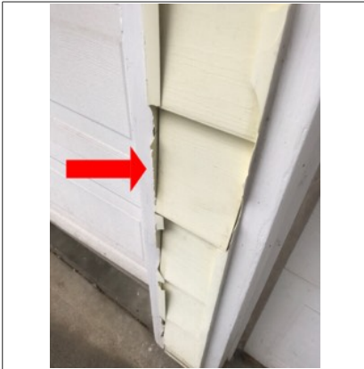
Multiple locations of exterior vinyl trim is chipped and broken
