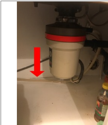
Dishwasher drain is not looped above underside of kitchen sink
